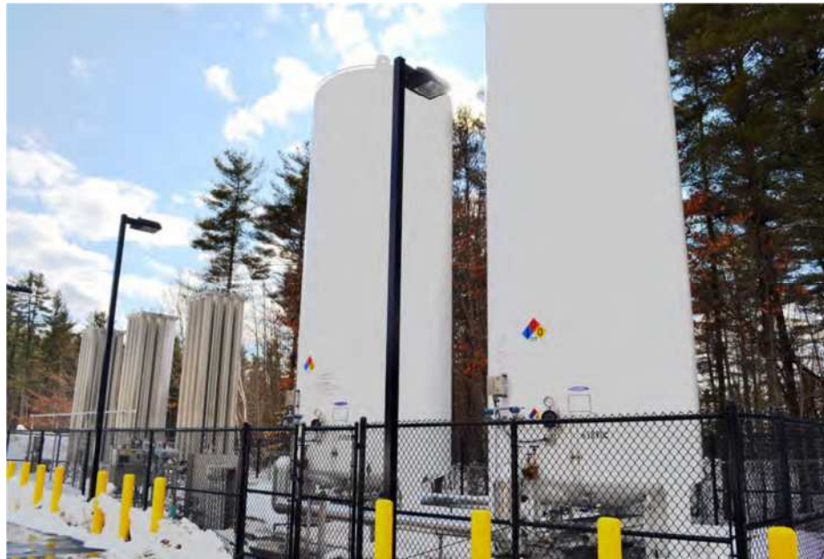
New Liquid Oxygen Storage System
