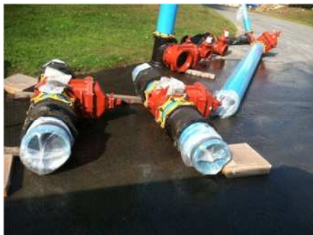
New 12 inch valves are preassemble to be installed on County Road in Westbrook
