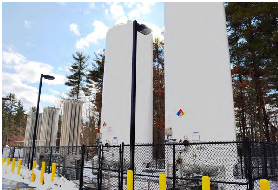
Liquid Oxygen Storage System
