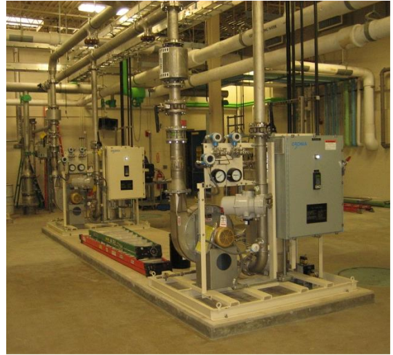
Managed Ozone Destruct System upgrade project
