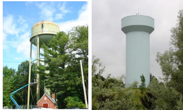
2018 – Design of elevated Storage for 407 zone north. This project will replace an old undersized 1950 Tank (left) with new tank (right)
