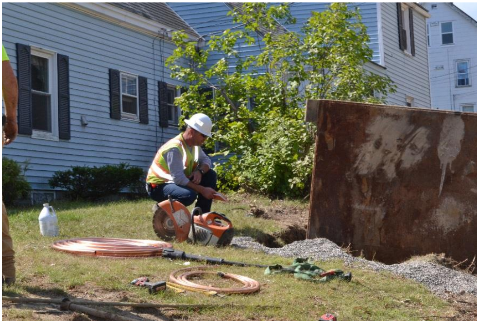
District's Water Utility Specialist Joe Gray inspecting a new water service installation on the Mitchell Street, Westbrook. The District replaced 400 feet of 8" cast iron 1955 vintage water main with a new 8" ductile iron water main on Mitchell Street as part of the Westbrook CSO separation project.
