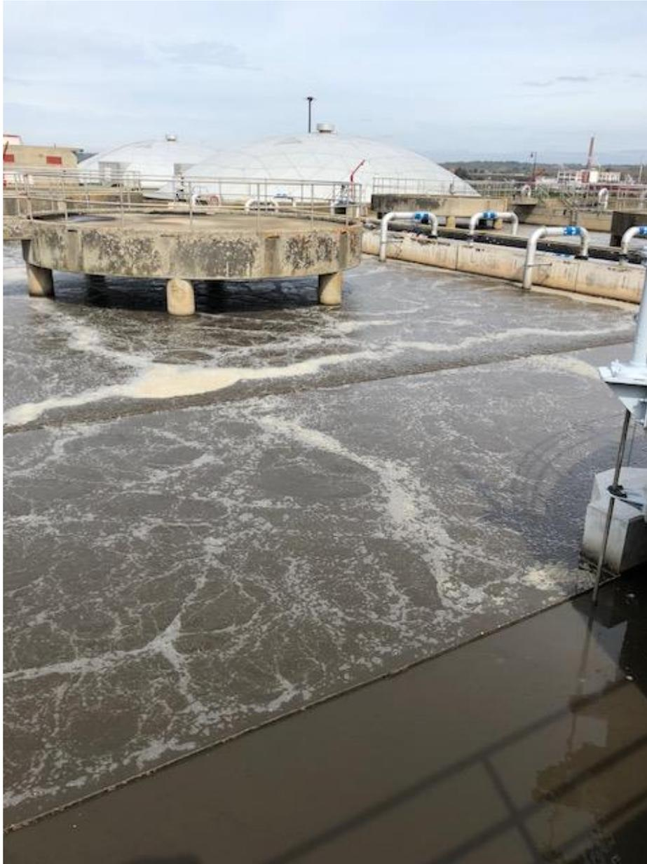
New diffused aeration system – note the mixing and air bubbles in the tank.
