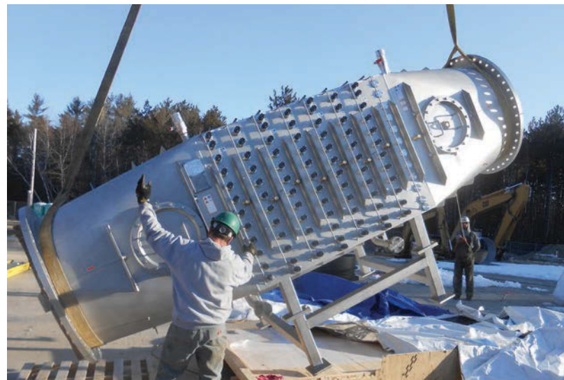
A UV reactor is delivered to the Sebago Lake Water Treatment Facility
