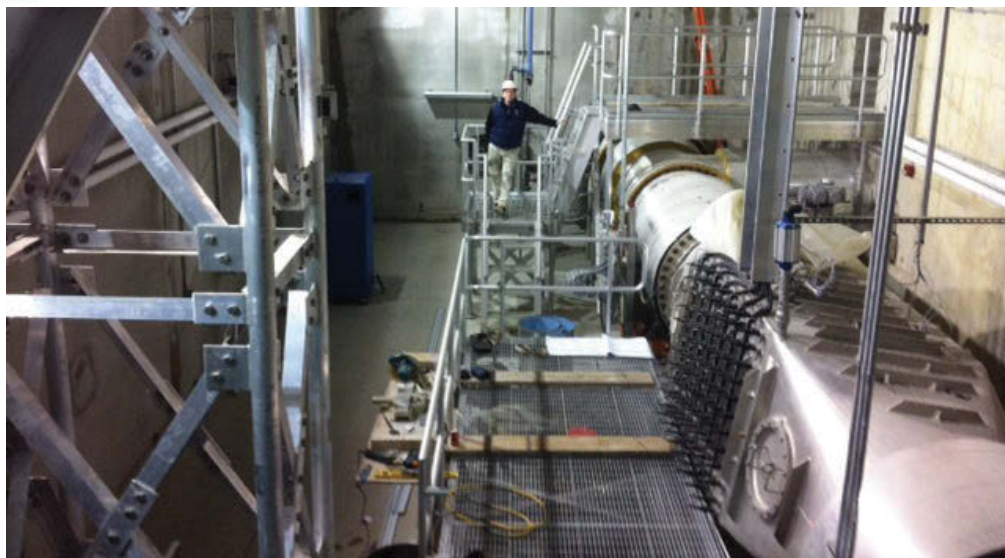
UV equipment installed inside the Sebago Lake Water Treatment Facility
