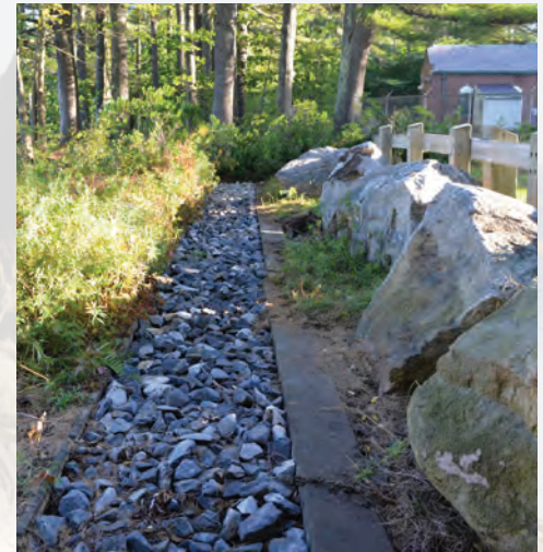
The stone was replaced in this infiltration trench at Chadbourne's Landing as part of the Sebago Lake Erosion Control Project.
